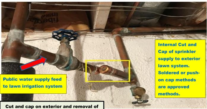
Cut and cap on exterior and removal of existing backflow preventer is required.
