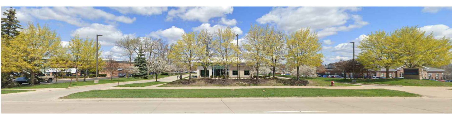
EXISTING CONDITION - SITE FRONTAGE NOT TO SCALE
