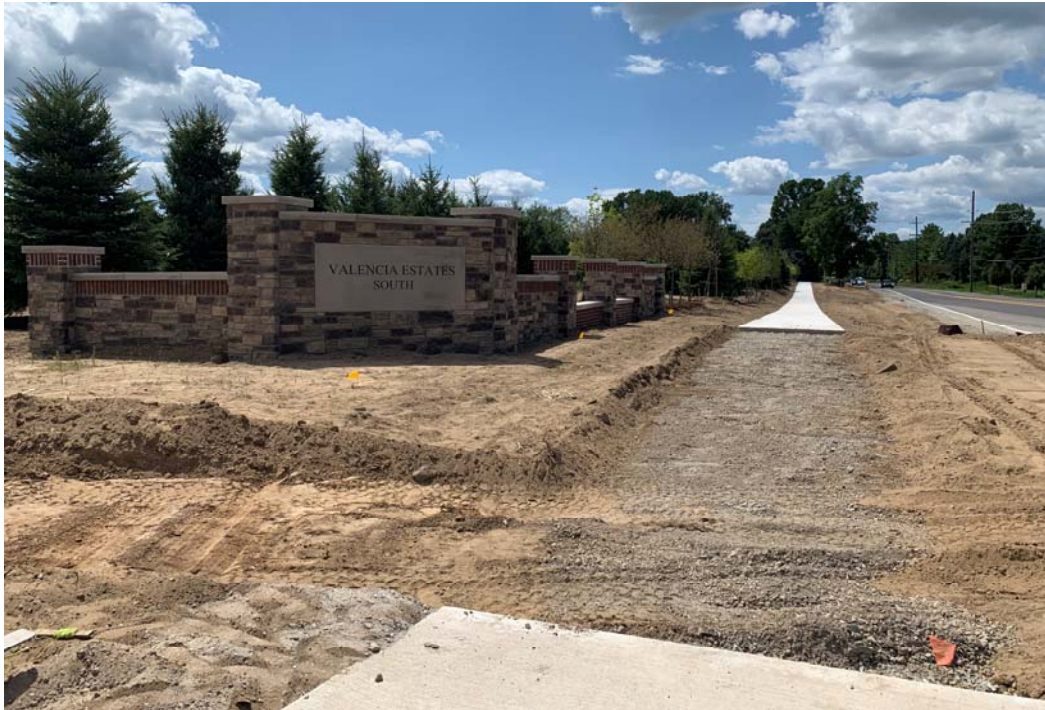
Segment 99b: Sidewalks built by Private Developers along Ten Mile Road
