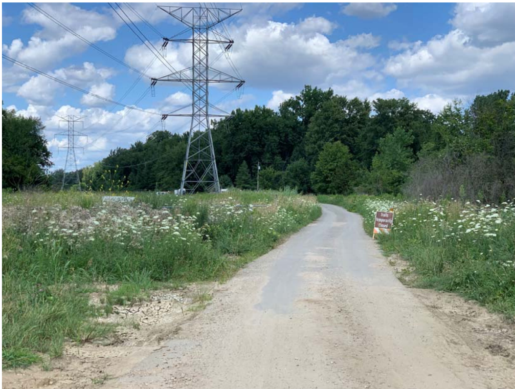
Under Construction: ITC Trail between Nine Mile Road and Ten Mile Road
