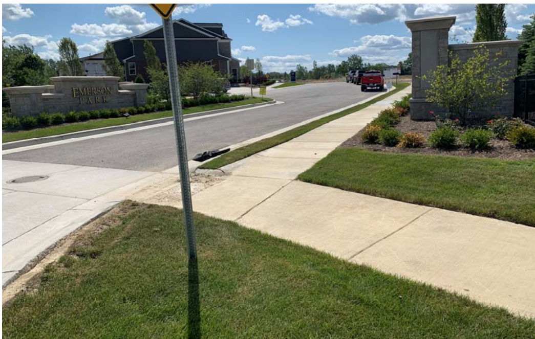
Existing sidewalk widened to 6 feet as part of Private Development along Novi Road
