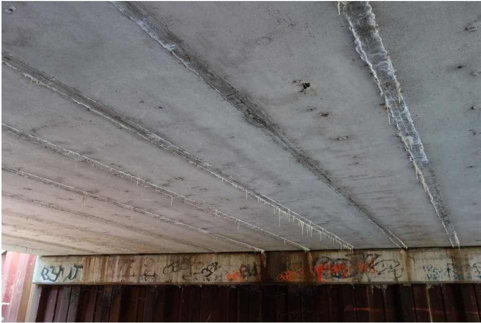
Typical Deck Underside
