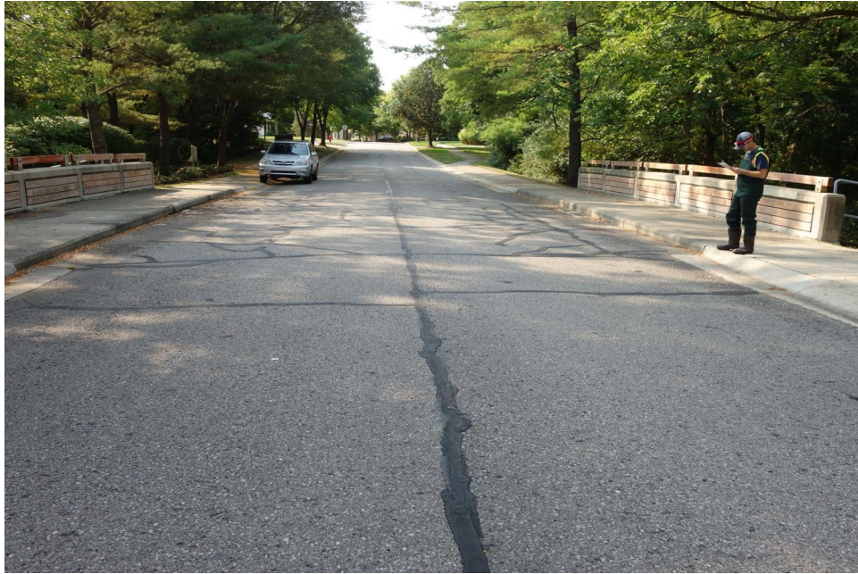
North Approach Looking South
