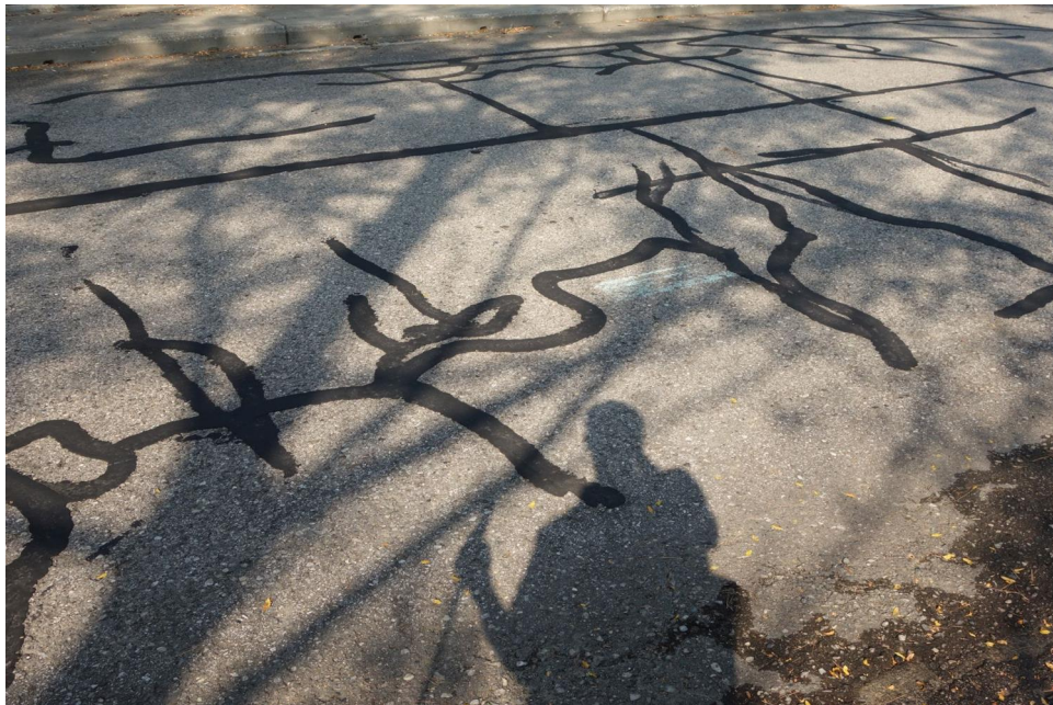
Typical Deck Surface
